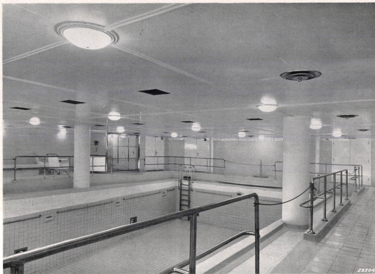
Fig. 9. The swimming pool of the "Nieuw Amsterdam" also has the low ceiling typical of ships. The plafonniers described in the text were used for the built-in illumination from above. By making the bowls of "Philippan" glass (see Philips techn. Rev. 3, 47, 1938) all the colours are deepened and the skin takes on a warm colour against the beautiful green of the pool.
