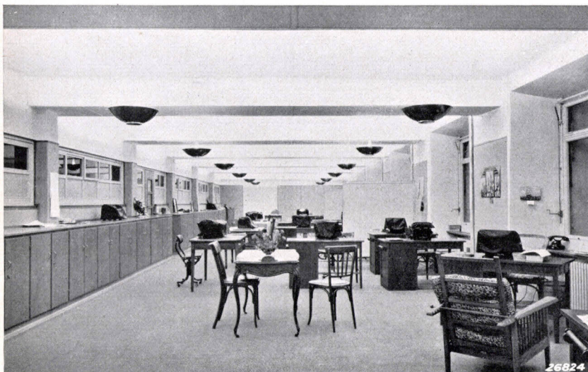
Fig. 4. Indirect illumination with WX fixtures; the placing of the desks is here independent of the lighting.
