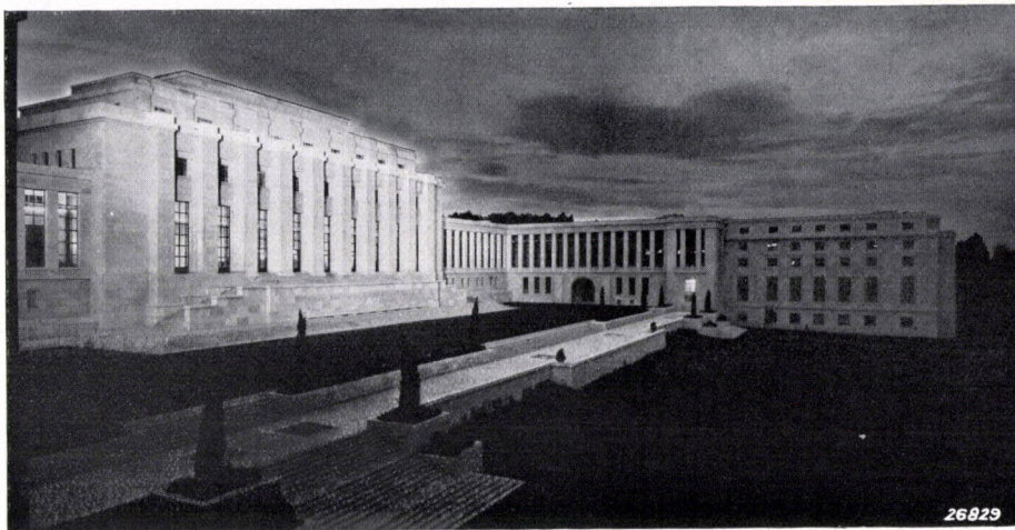
Fig. 14. Lighted exterior giving on the "Cour d'Honneur".
