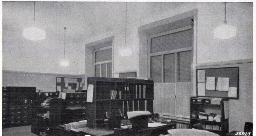
Fig. 3. Illumination with diffusing fixtures DM of one of the rooms of the secretarial department of the League of Nations.
